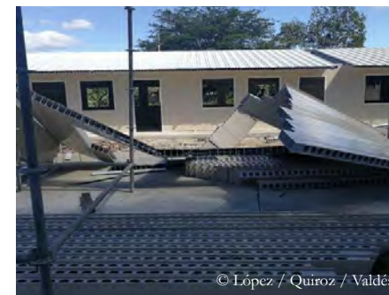
Margarita Maza de Juárez school post-earthquake reconstruction
